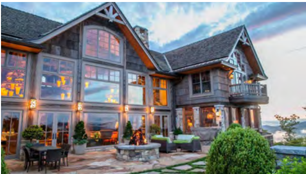
▲ The Spa at Old Edwards Inn, Highlands, NC
